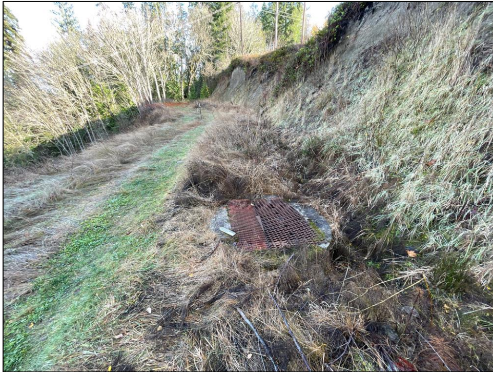
Figure 6.2-6. Highland Canal, Feature 2, showing the concrete enclosure with access to the piped portion of the canal under the BPA transmission line ROW.
