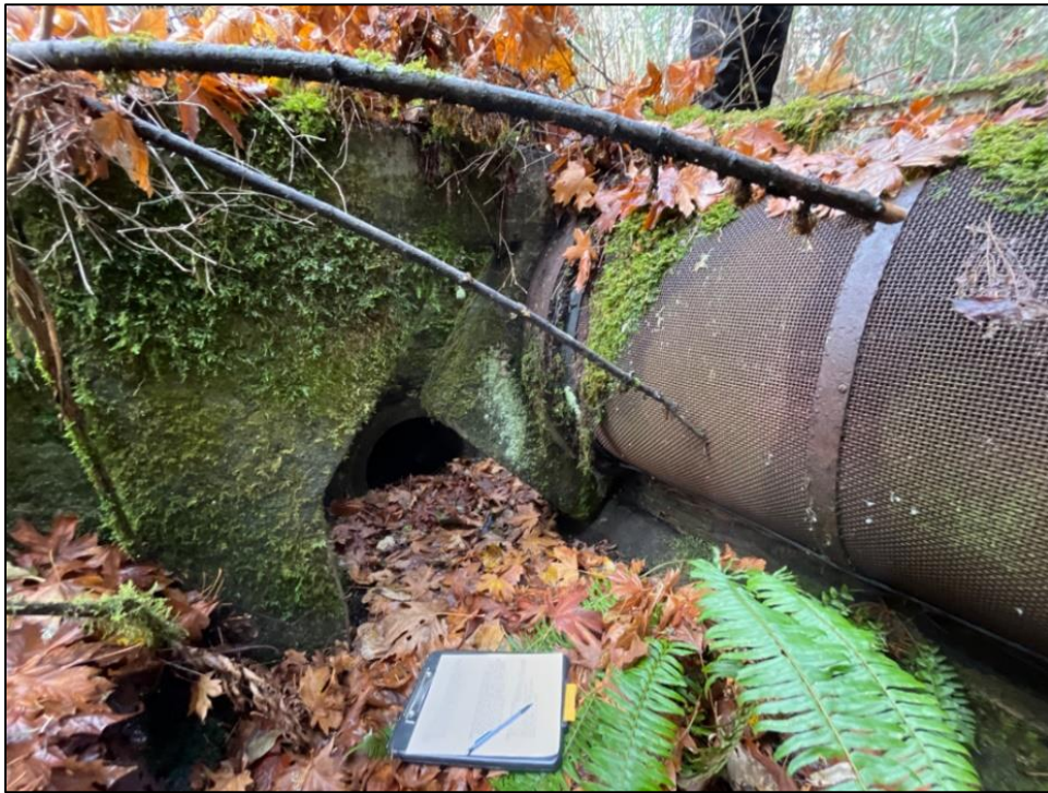
Figure 6.2-19. Independent Intake Canal, Feature 2, showing rotating drum trash screen and culvert outlet, looking northwest.
