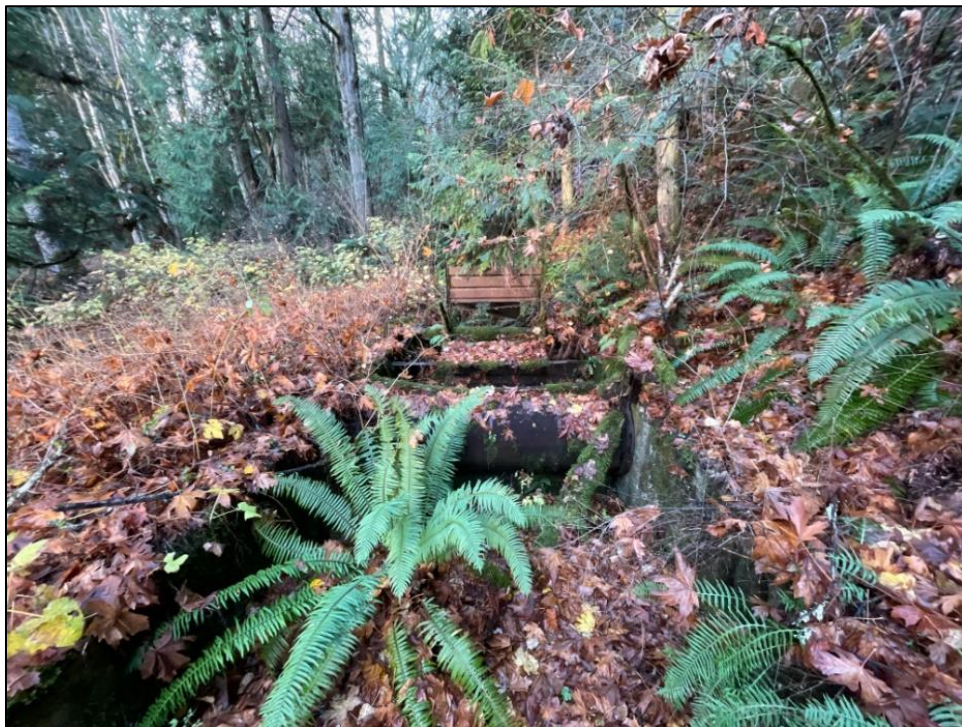
Figure 6.2-17. Independent Intake Canal, Feature 2, showing the trash screen mechanism and concrete-lined walls of the abandoned ditch, looking northeast.
