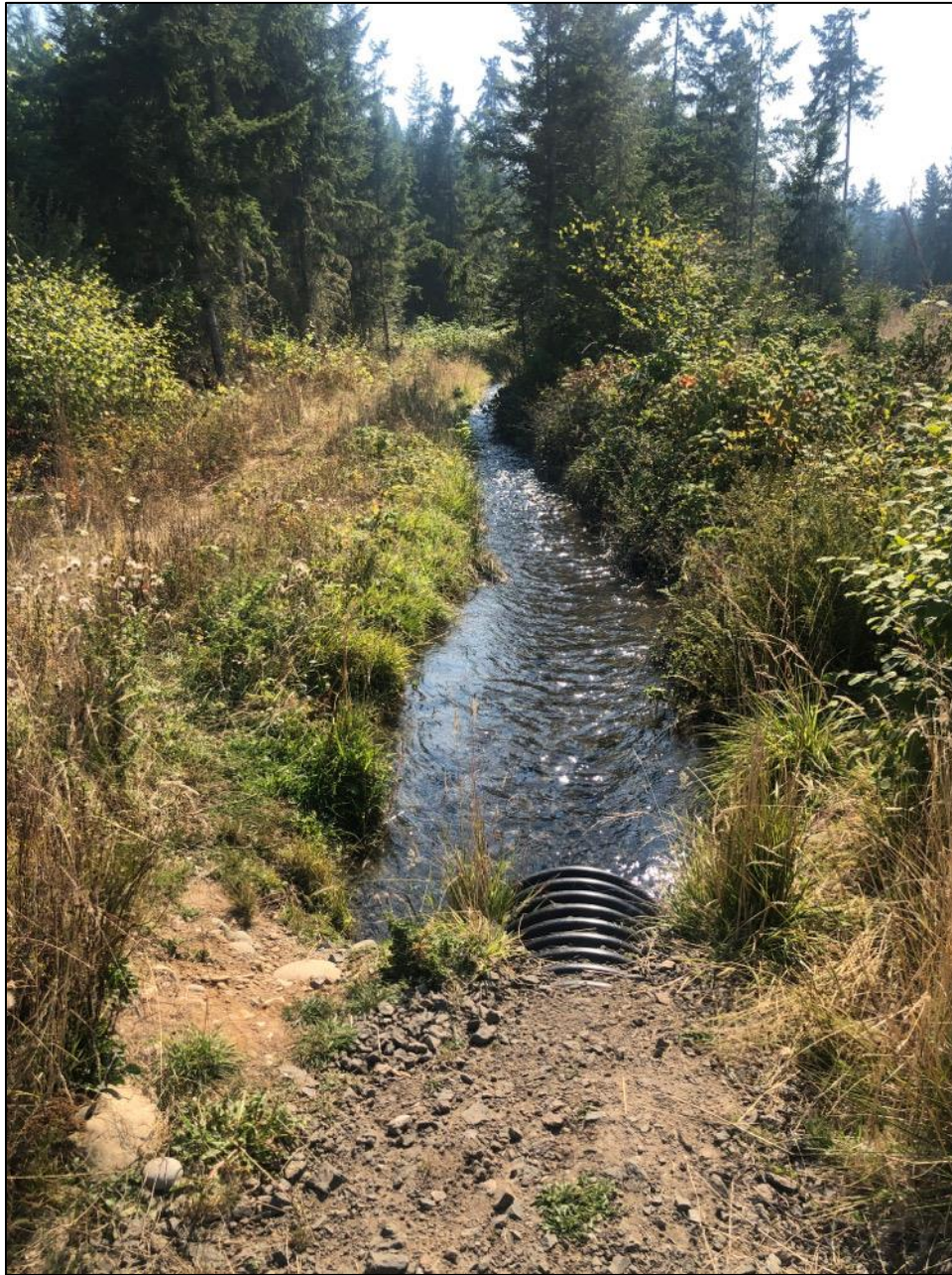
Figure 6.2-9. HC-1 Lateral of the Highland Canal, Feature 4, showing plastic culvert under access road within BPA transmission line corridor, looking south.
