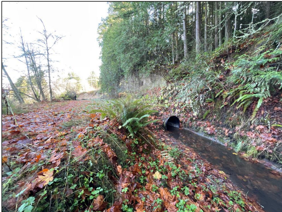
Figure 6.2-5. Highland Canal, Feature 2, showing the southwest end of the plastic culvert pipe channeling the Highland Canal under ground within the BPA transmission line ROW; looking northeast.
