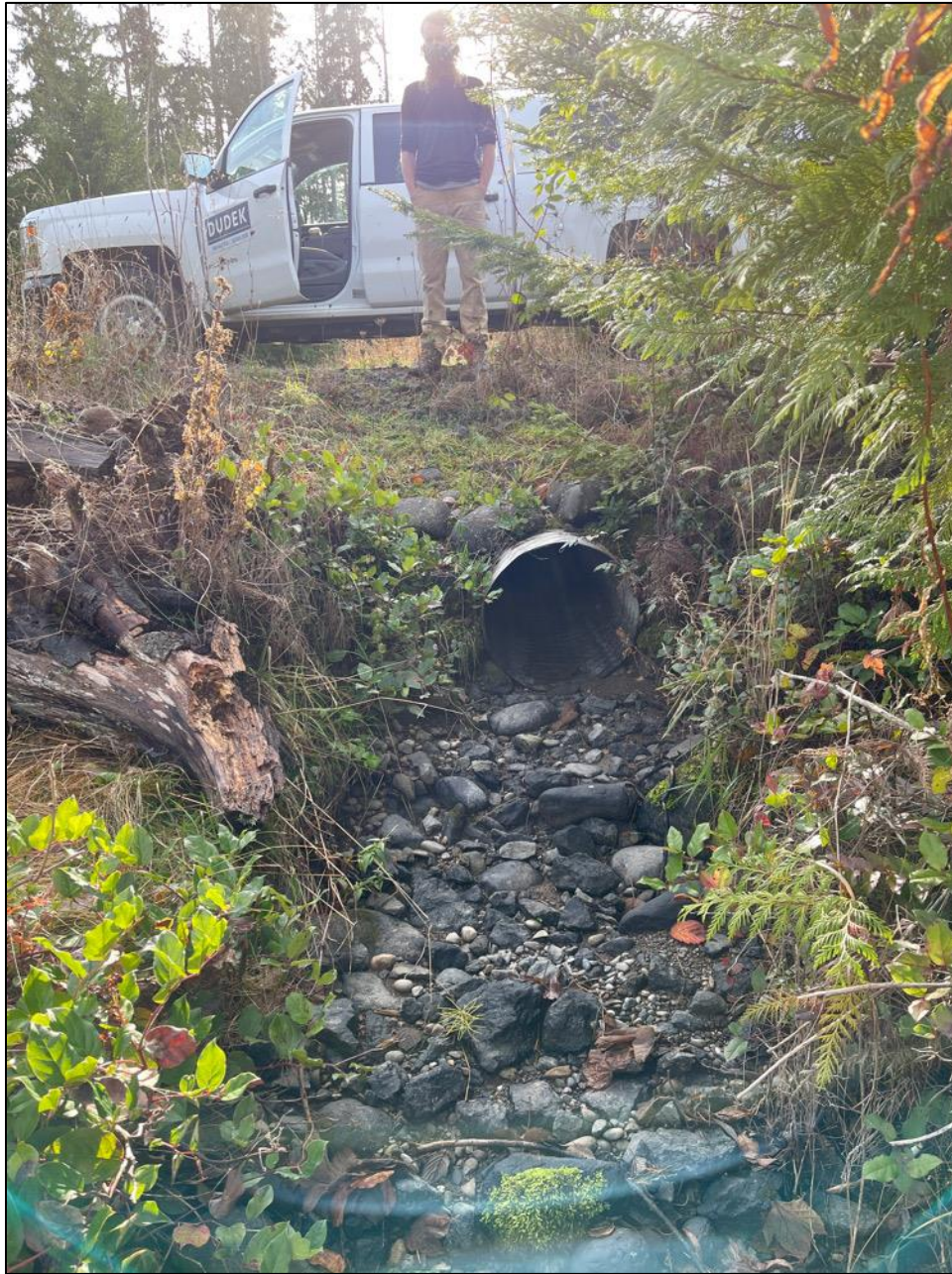
Figure 6.2-10. HC-1 Lateral of the Highland Canal, Feature 5, showing metal culvert under access road within the proposed reservoir area, looking south.
