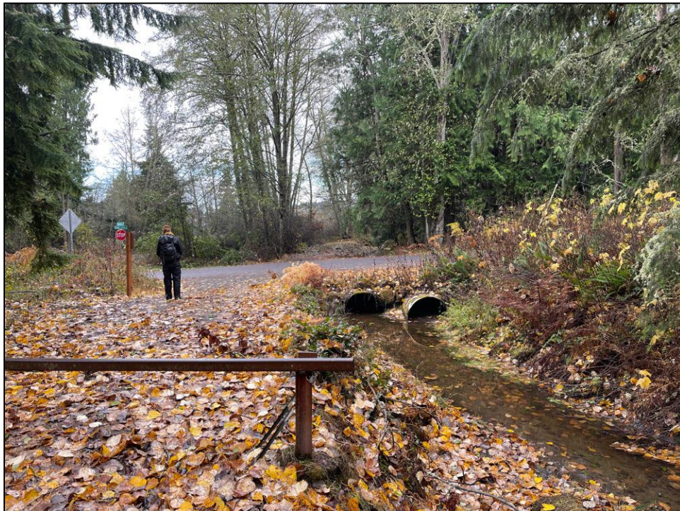
Figure 6.2-7. Highland Canal, Feature 3, showing double culvert pipes beneath Sporseen Road.
