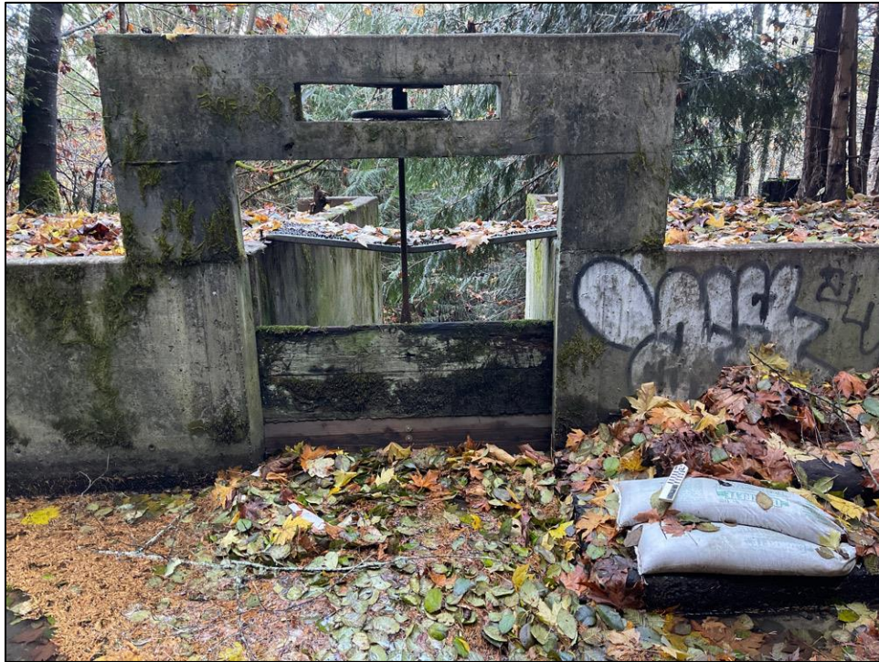
Figure 6.2-4. Highland Canal, Feature 1, showing the metal gate and spillway beyond, looking west. Leaves cover the surface of the water in the canal ( foreground ).
