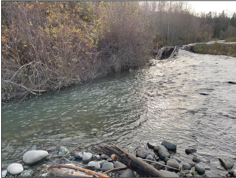
Figure 6.2-14. Independent Intake Canal ( left , flowing toward bottom left of photo) showing the diversion point at side channel of the Dungeness River ( right ) and concrete escarpment at bank ( background center under brush) preventing bank erosion, looking southeast.
