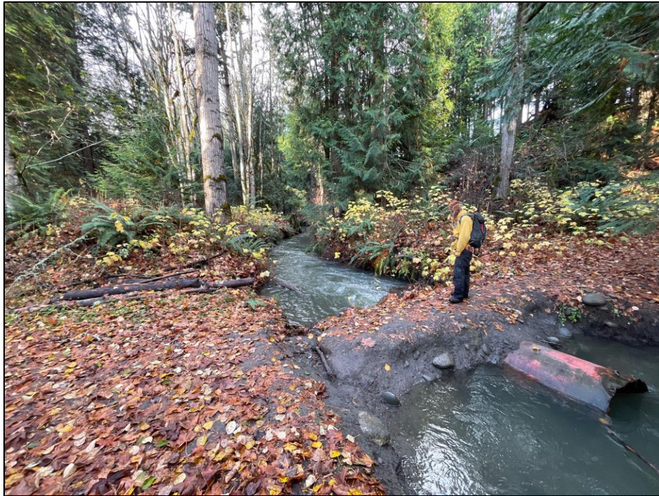
Figure 6.2-16. Independent Intake Canal, Feature 1, showing culvert pipe and berm for pedestrian trail, looking northeast.
