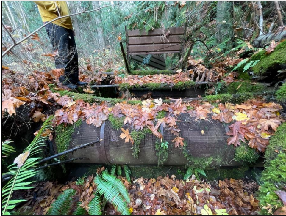
Figure 6.2-18. Independent Intake Canal, Feature 2, detail view of trash screen and paddle wheel, looking northeast.
