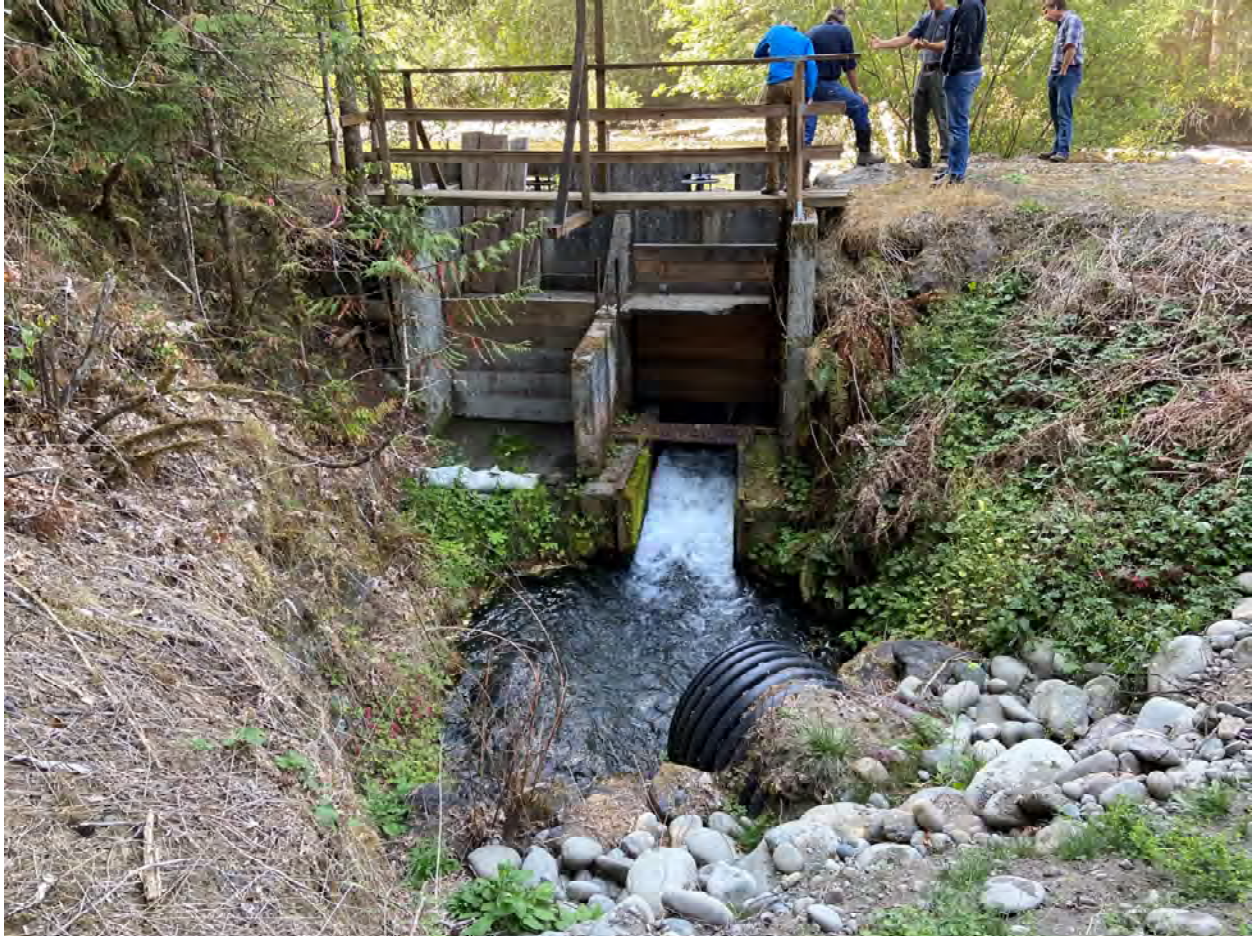
Figure 3 Highland Ditch Diversion Headgate (Two - 3 ft wide by 3 ft tall unseating head mounted slide gates)
