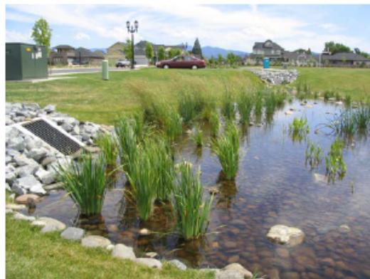
Figure 2: Wet swale detention facility
