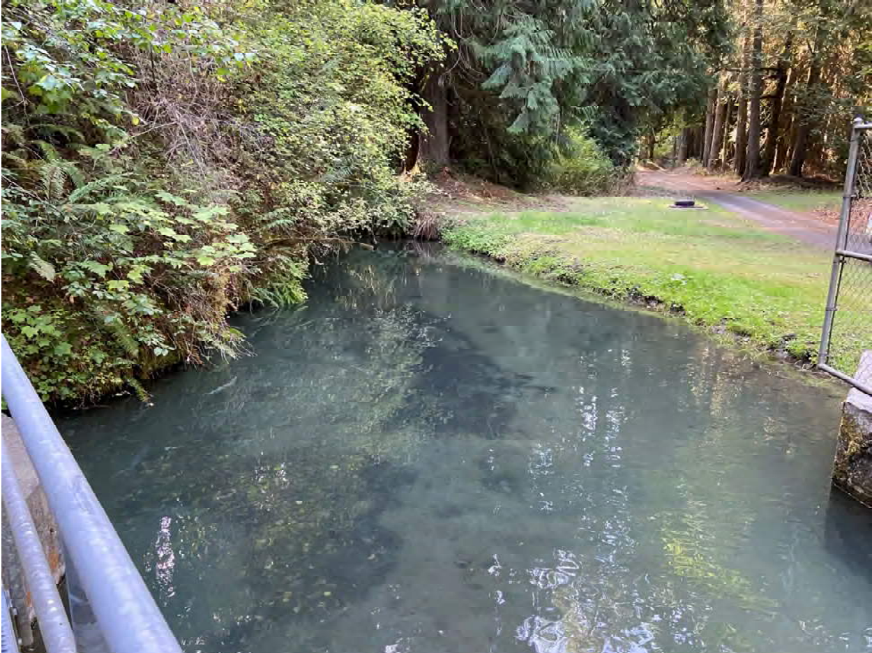
Figure 5 Highland Diversion Ditch Canal just upstream of Diversion Structure
