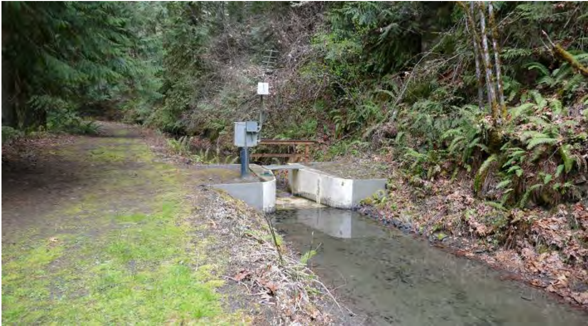
Photograph 12 Parshall Flume at Upstream End of HID Main Canal Downstream of Fish Screens
