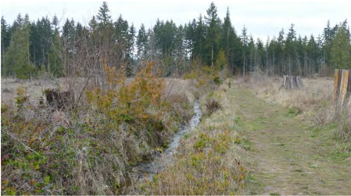
Photograph 3 H1 Lateral and Access – Near North End of Site Looking North
