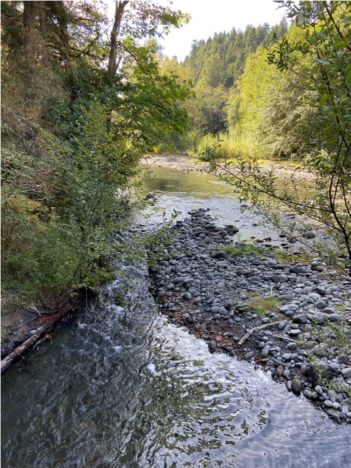
Figure 1 Right bank diversion channel off the Dungeness River at River Mile 11.0
