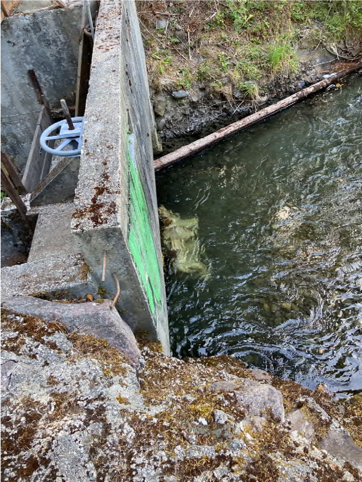
Figure 2 Upstream concrete face of Highland Diversion Ditch Headgate
