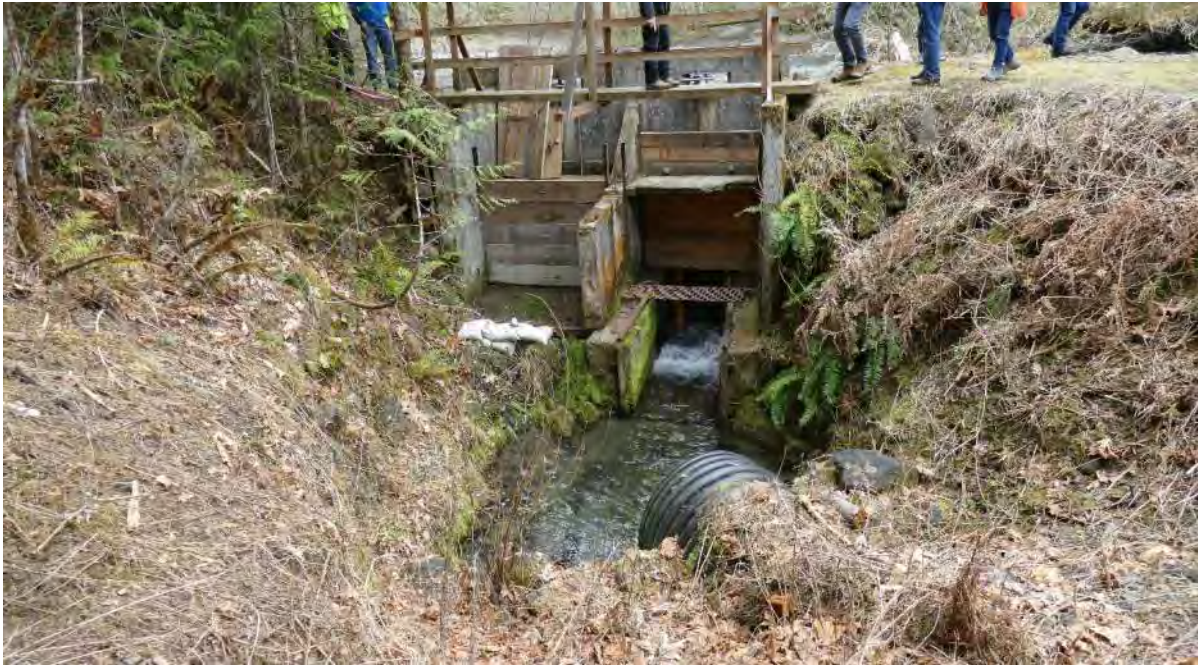
HID Headgates and Intake Structure on Dungeness River (From Downstream Side)
