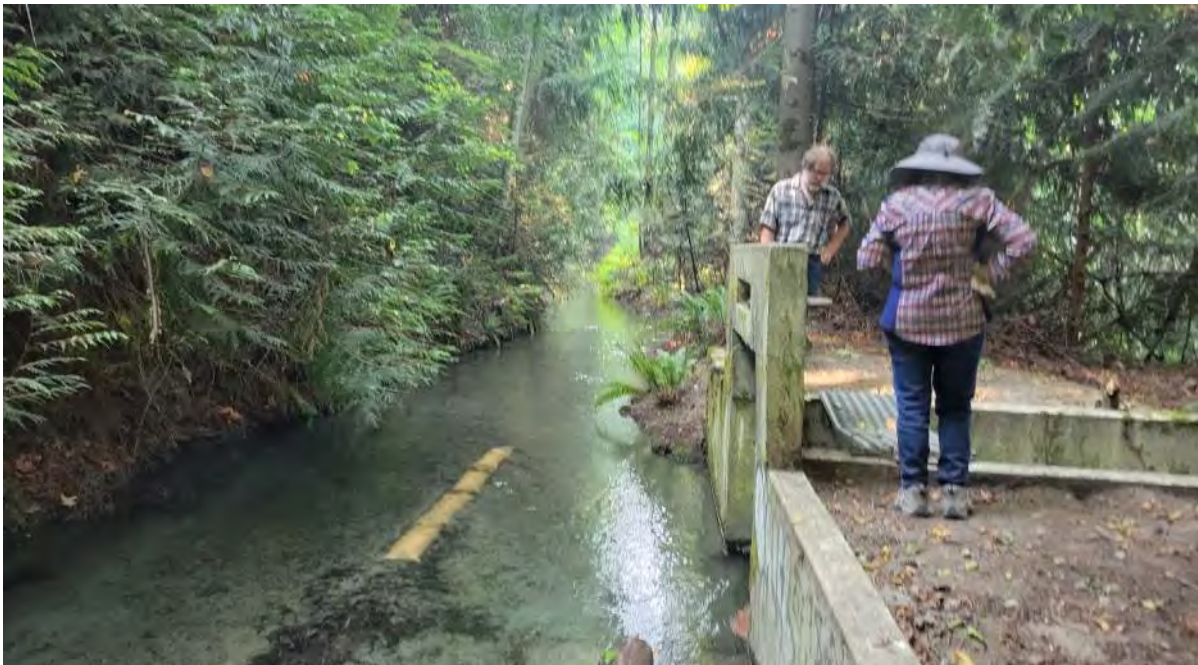
Photograph 14 H1 Lateral Inlet Structure on HID Main Canal
