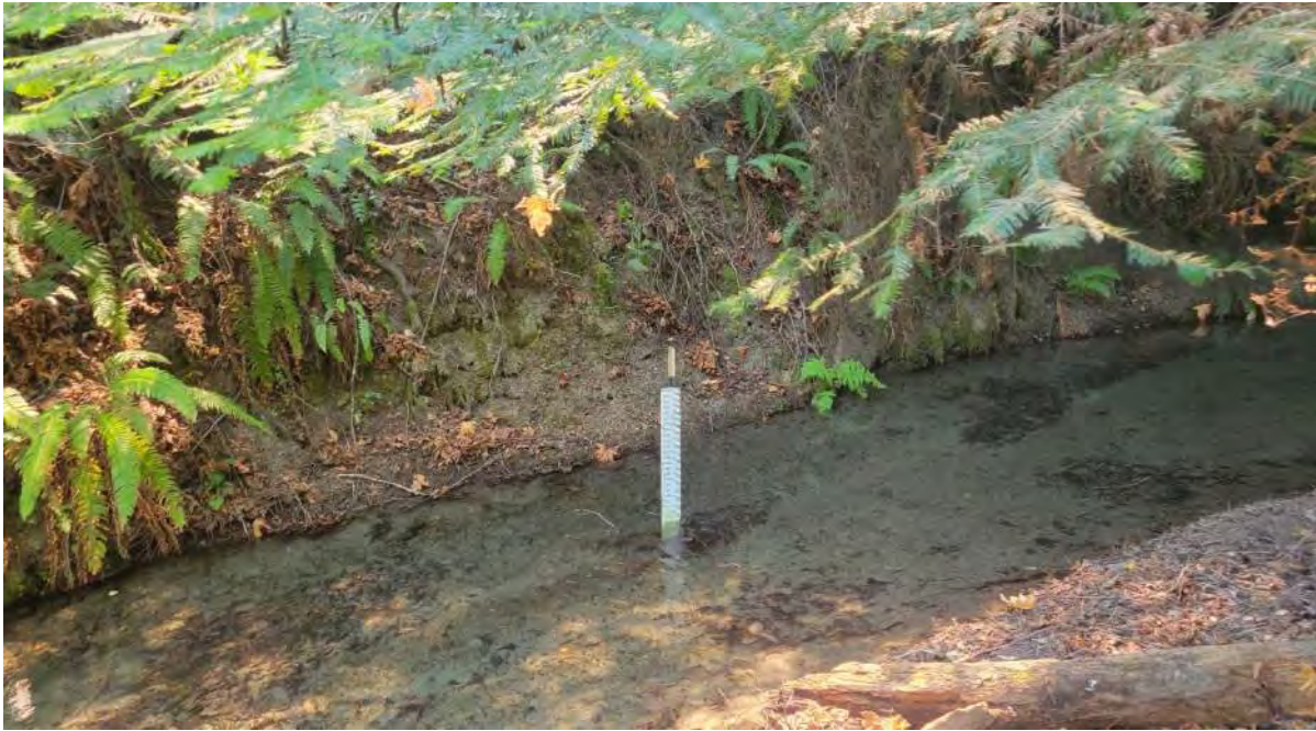
Photograph 15 HID Main Canal Downstream of H1 Lateral Structure
