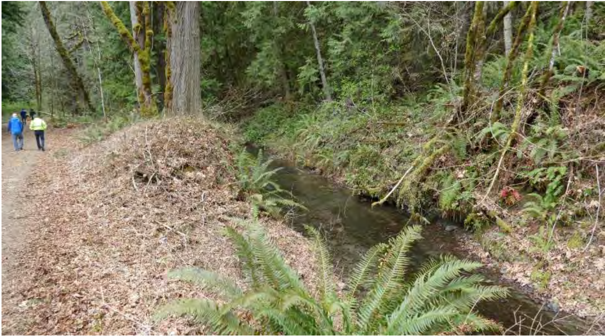
Photograph 13 HID Main Canal Downstream of Fish Screens
