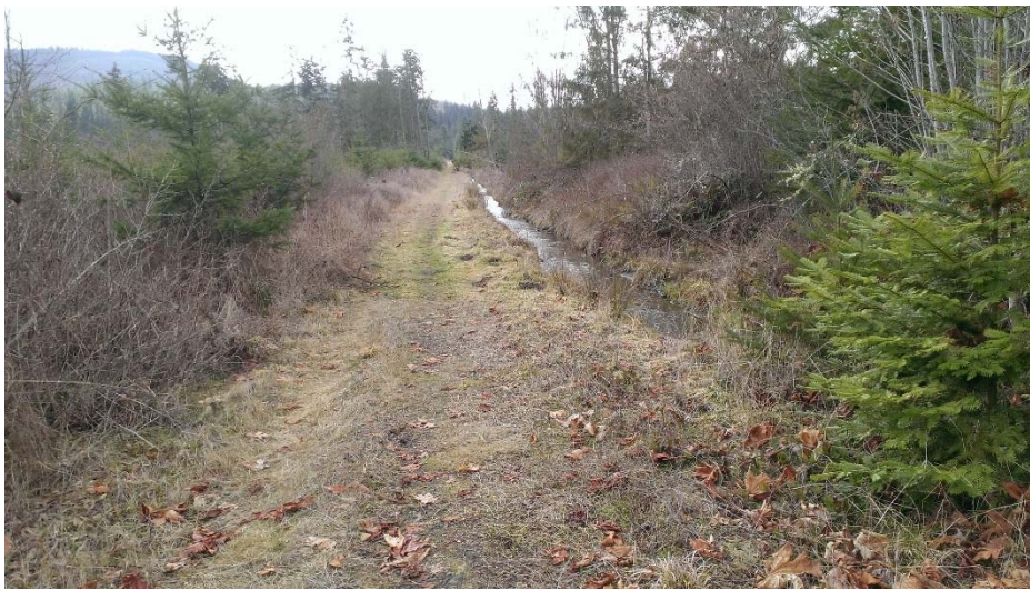
PHOTOGRAPH 2 Dungeness Off-stream Storage Site from approximate location of proposed reservoir outlet looking south along the HID lateral. The lateral bisects the site, flowing south to north.
